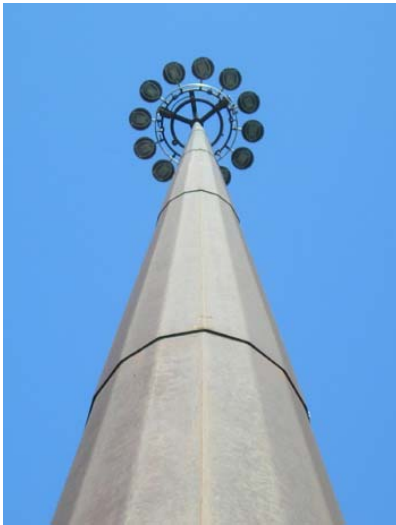
Figure 4.38 Typical High-Mast Luminaire Structure (Road Traffic Technology Lighting Solutions Image Gallery n.d.)
