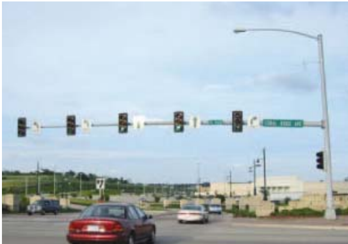
Figure 4.1 Typical Mast-Arm Structure
