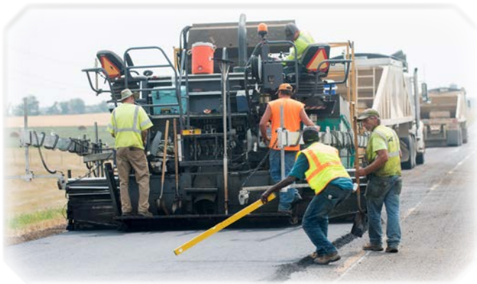
Resurfacing a highway in Dickinson District.
