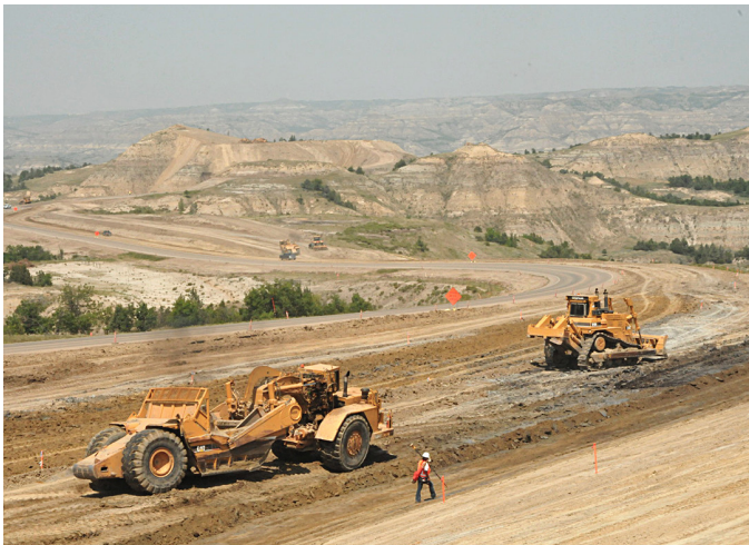
2011 construction work on ND Highway 22 north of Killdeer
