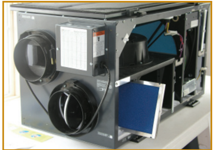
Figure 13-B. Filters in a heat exchanger. (Photos courtesy of Shirley Neimayer, University of Nebraska - Lincoln).
