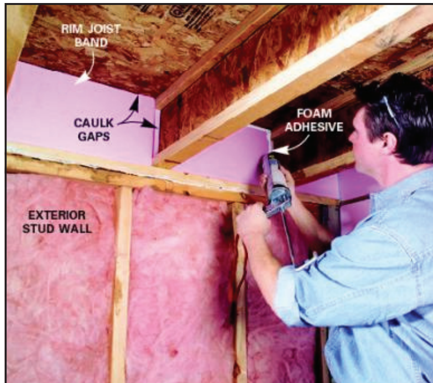
Figure 7. Insulating the rim joist and sealing air leaks with rigid insulation. Insulation needs to be covered with a 15-minute fire barrier.
