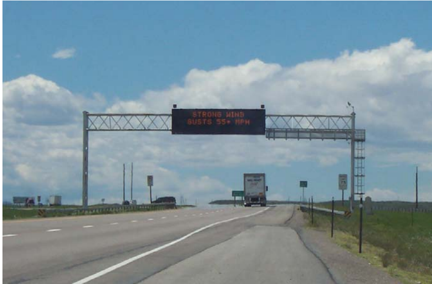
Figure 3.3 Three-line Overhead DMS at milepost 356.7, westbound
