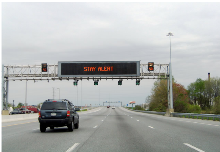
Figure 2.1 Overhead dynamic message sign
