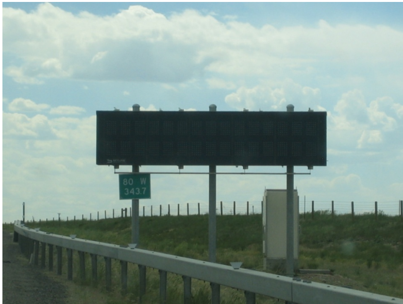
Figure 3.5 Two-line Sidemount DMS at milepost 343.7, westbound
