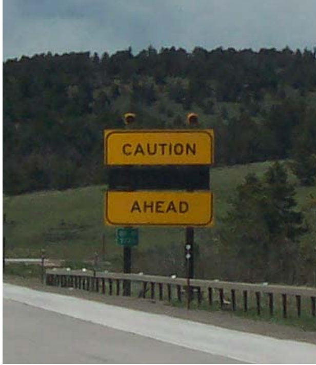
Figure 3.4 One-line Blank-Out DMS at milepost 322.6, westbound
