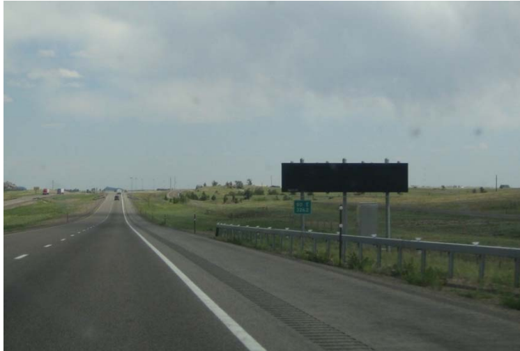
Figure 2.2 Roadside dynamic message sign
