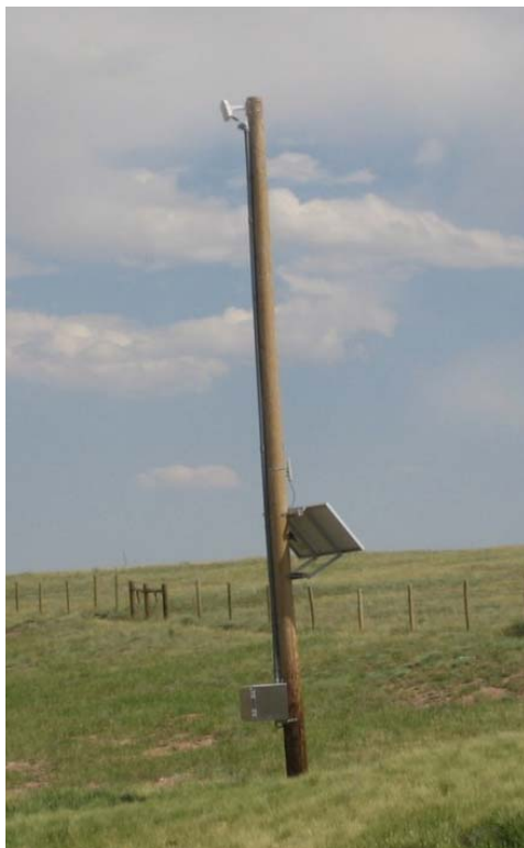
Figure 3.6 Speed sensor at milepost 330
