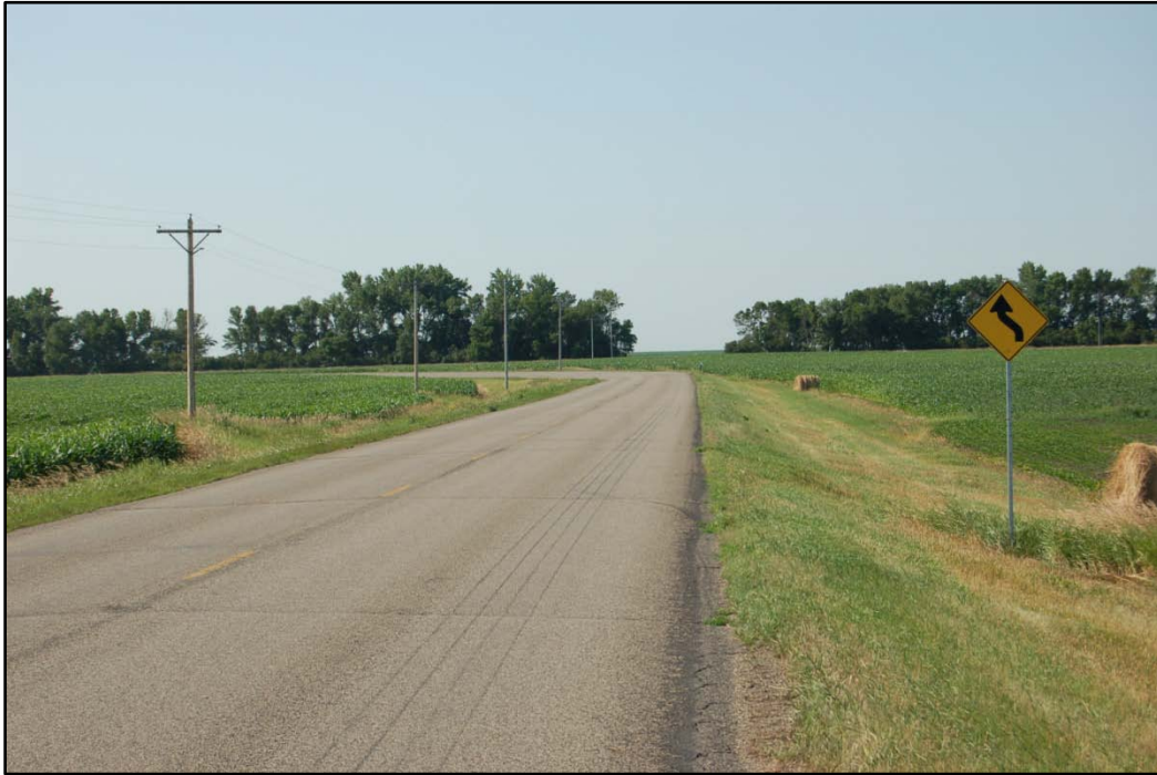
Figure 5.1 Horizontal curve north of Valley City
