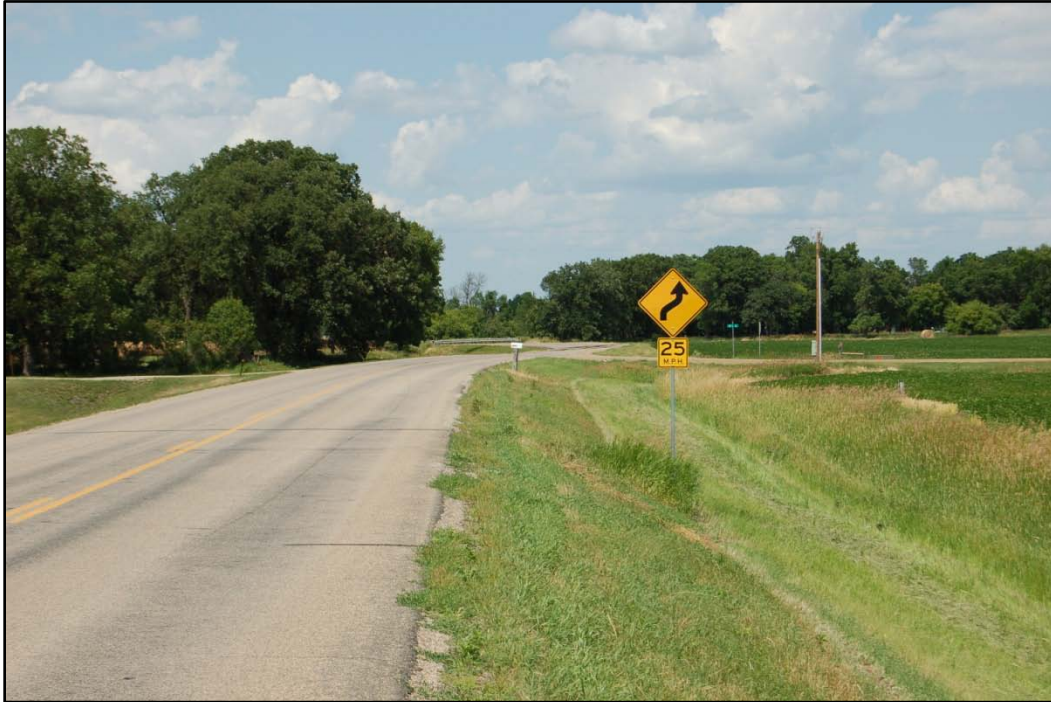
Figure 5.7 Bridge and horizontal curve south of Valley City, N.D.
