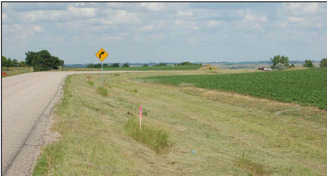
Figure 5.19 Large horizontal curve on Highway 21
