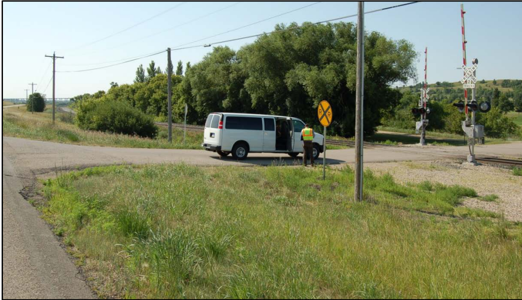
Figure 5.6 Railroad crossing northwest of Valley City, N.D.
