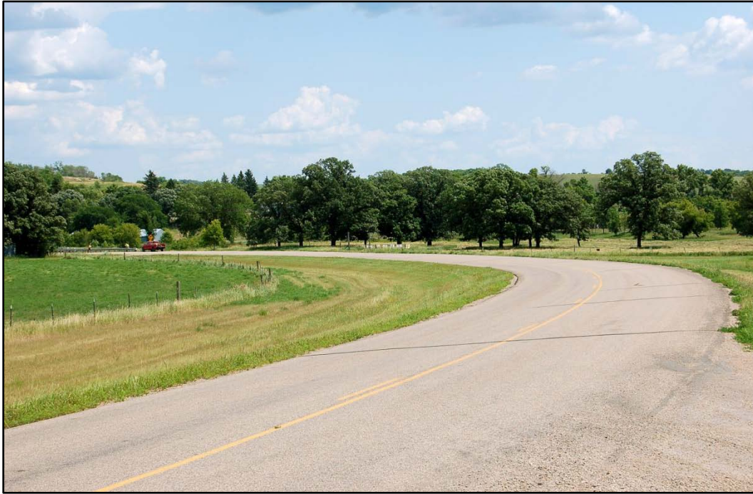
Figure 5.8 North end of Skorpen Curve Note: Photo was taken facing to the southeast
