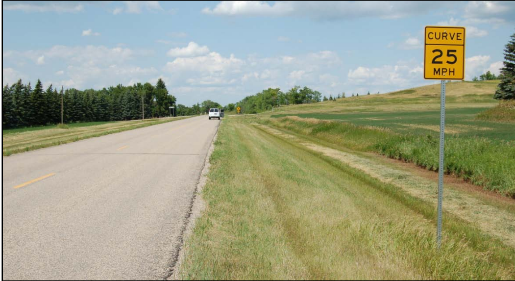
Figure 5.12 Advanced speed advisory sign (northbound at Skorpen Curve)
