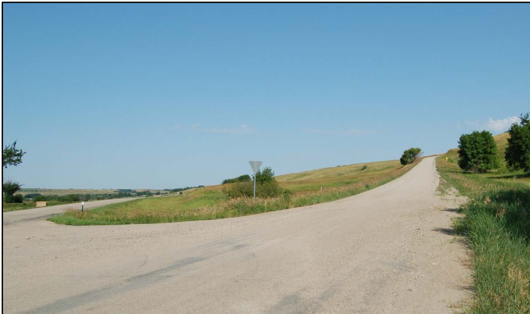
Figure 5.5 Obstruction and alignment issues at the Bloomberg Hill intersection
