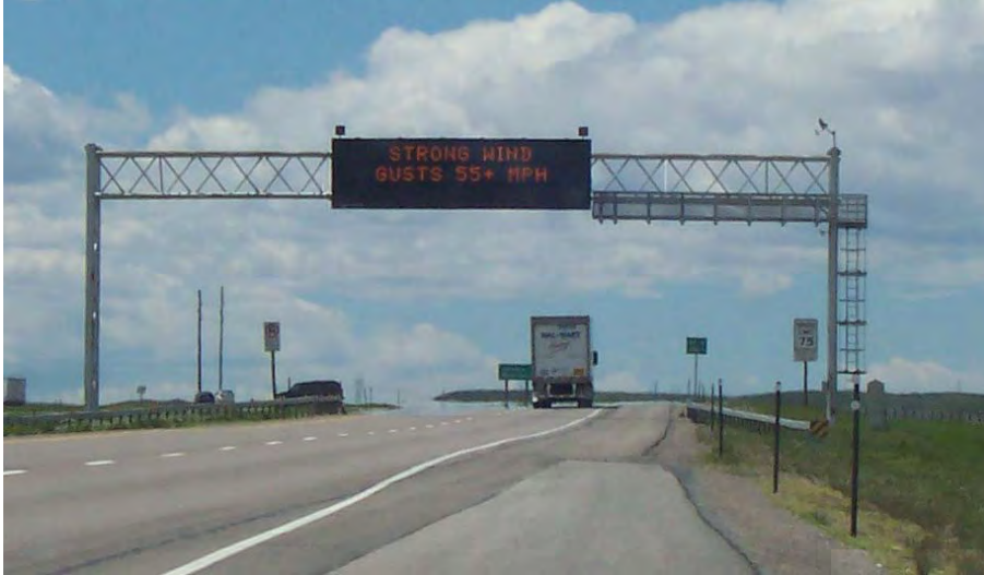
Figure 2.3 Three-line Overhead DMS at Milepost 356.7, westbound
