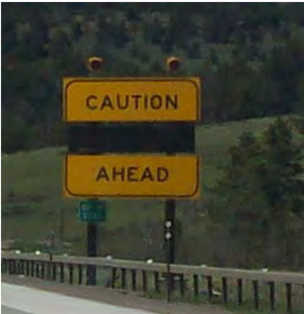
Figure 2.4 One-line Blank-Out DMS at Milepost 322.6, westbound
