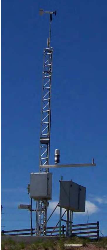
Figure 2.7 RWIS Station at Milepost 329.4
