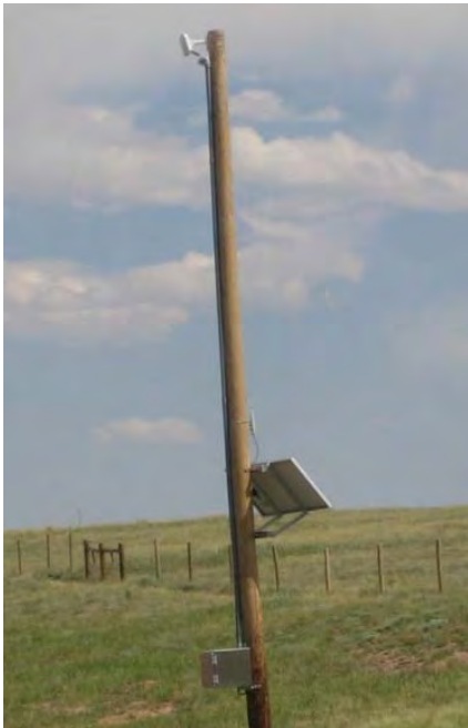
Figure 2.6 Speed Sensor at Milepost 330
