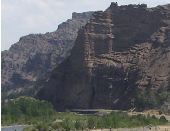
Figure 4.27 Hanging Rock Section Retaining Wall
