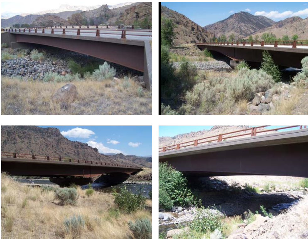
Figure 4.26 Hanging Rock Section Bridges Clockwise from upper left: Clocktower Creek (MP 24.84), Elk Fork (MP 22.05), North Fork Shoshone River (MP 20.31), Clearwater Creek (MP 19.74).
