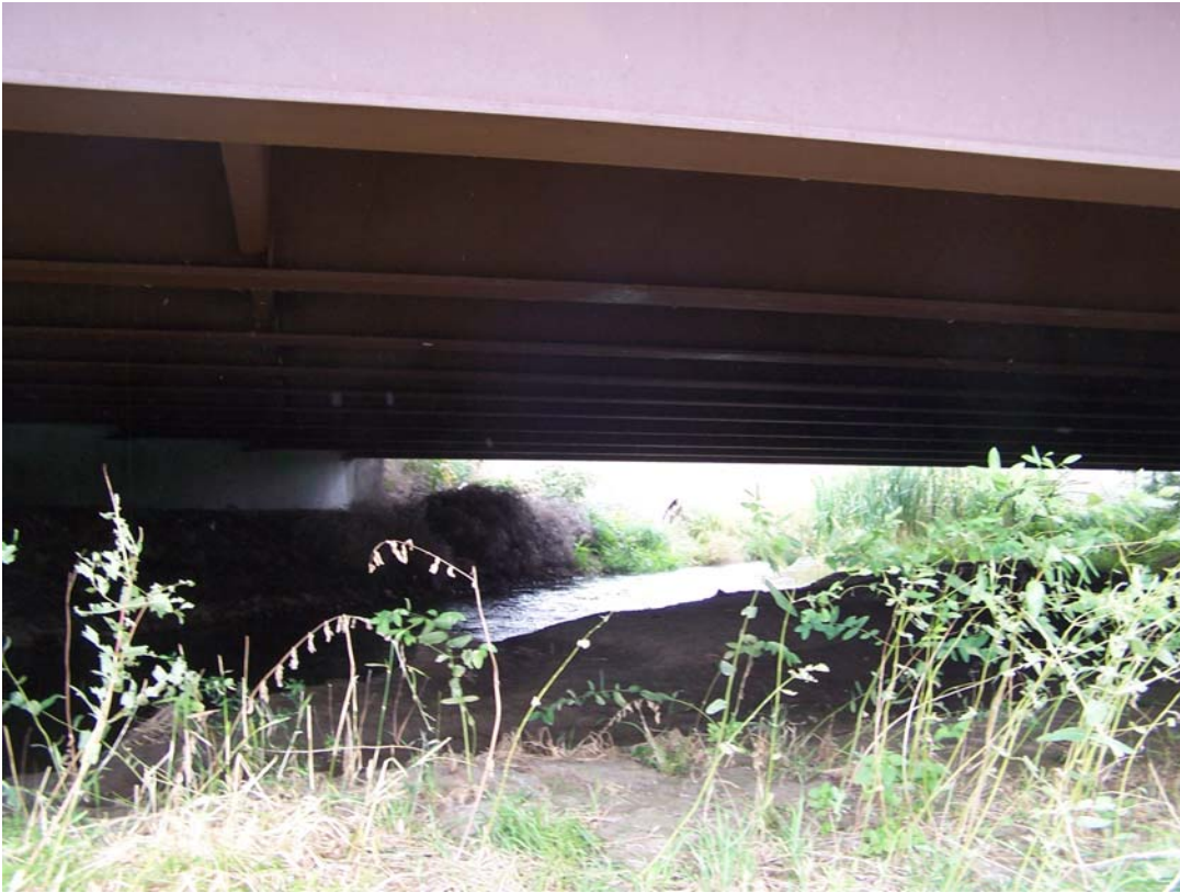
Figure 4.48 Rawhide Creek Bridge
