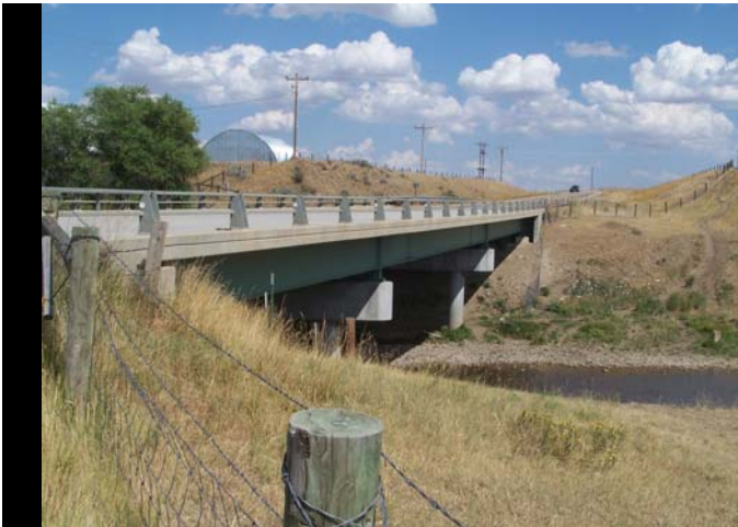
Figure 4.18 Clear Creek Bridge
