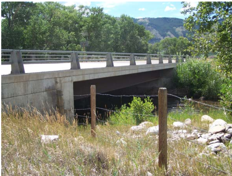
Figure 4.3 North Fork Little Laramie Bridge
