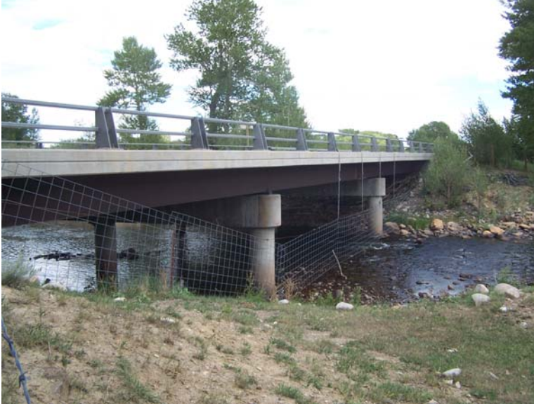
Figure 4.4 Little Laramie Bridge
