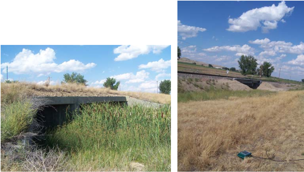
Figure 4.19 Culvert and Railroad Bridge at Creek Crossing
