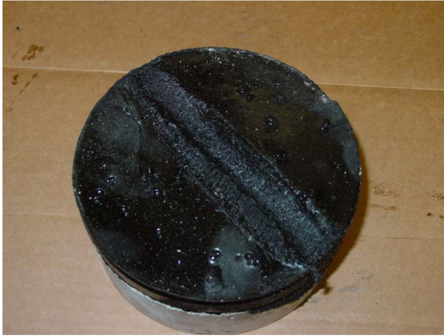
Figure 5.14 Rutting in PolyPatch Crack Surfacing Material
