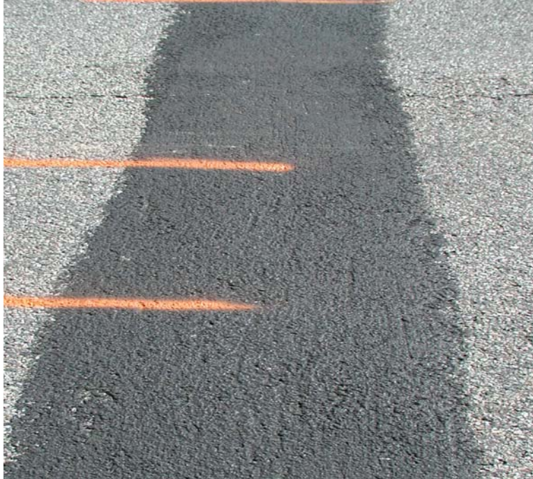
Figure 4.9 I-25 (MP 74.832) No Failure, Excellent Performance Throughout Traveled Way
