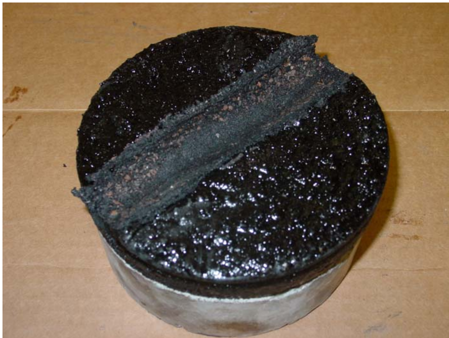
Figure 5.13 Rutting in Recessed Repair Mastic Crack Surfacing Material
