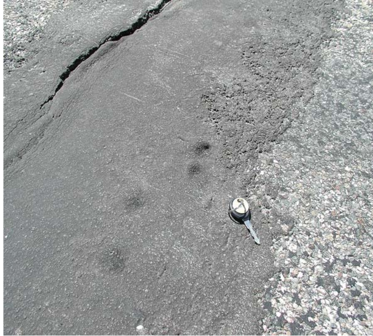
Figure 4.5 WY-93 (MP 25.554) Bubbling and Weathering Effects
