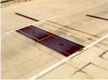
Figure 4.12: A Load Cell WIM System
