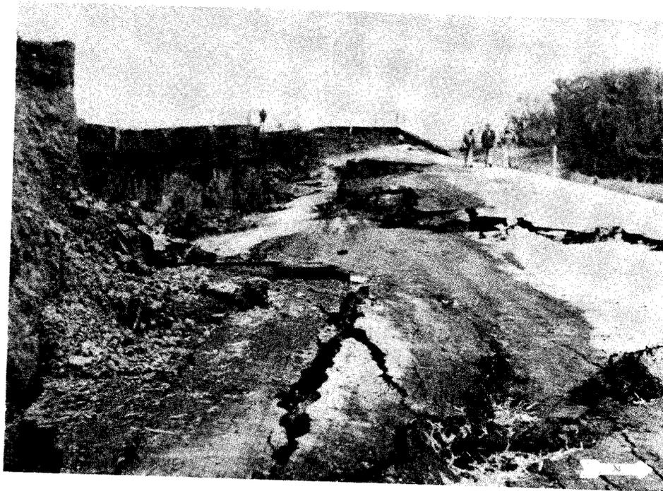
**Figure 30.** Photo of landslide that occurred several years ago on State Highway 17 at the Red River (NE  $\frac{1}{4}$ , Sec. 24, T. 157 N., R. 51 W.). This newly completed stretch of highway slid when the weight of the roadbed was too great for the weak, underlying clay unit to support. Photo by Robert L. Hetzler. (Bliss and Laird, 1963).
