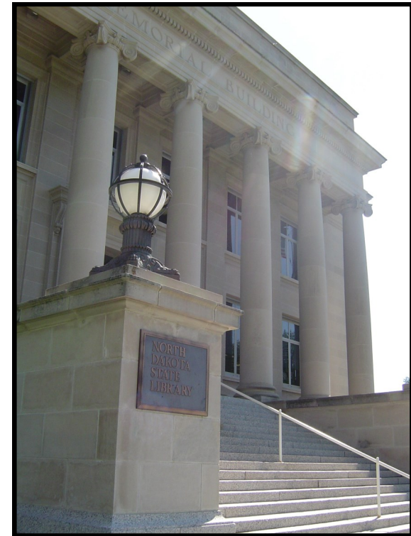
Liberty Memorial Building, Capitol Grounds, Bismarck, North Dakota.
